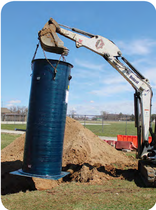
Lift Stations are also available in Vinyl Ester Resin for high temperature and corrosion resistant applications
